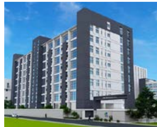
Figure: 360° TSL proudly achieved 1 more LEED Platinum Certificate for the DBL Group project.
